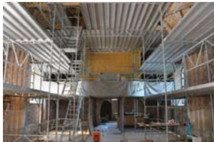
Scaffolding for the job of cleaning the paintings.
