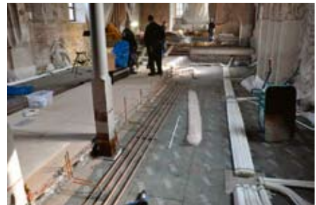
Installation of under-floor heating.
